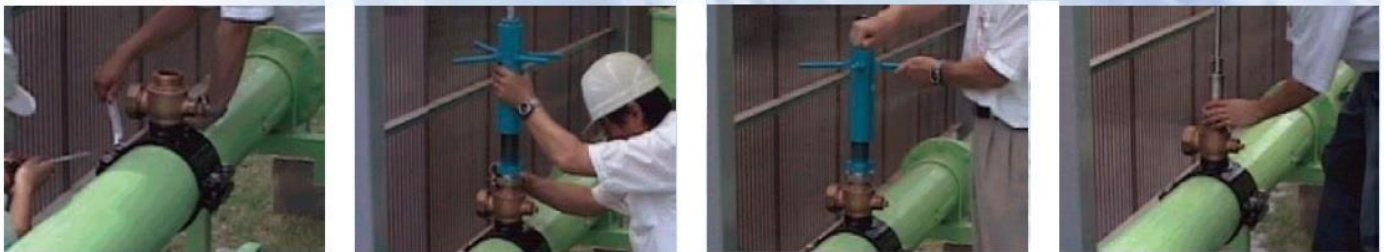
①The saddle points hydrant fixed on a pipe
