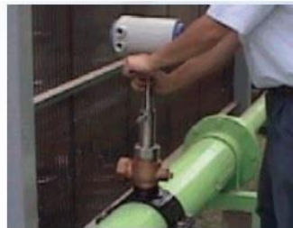
⑥:The flow meter is inserted into the pipe
